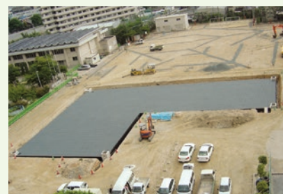
Elementary school in Fukuoka Prefecture 800m 3
