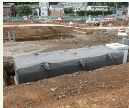
Town development in Saitama Prefecture 15m 3 ×140 subdivisions
