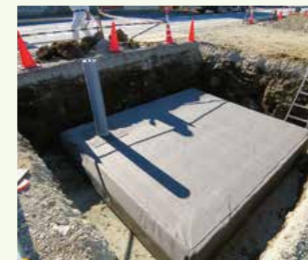
Housing land development in Saitama Prefecture 5m 3
