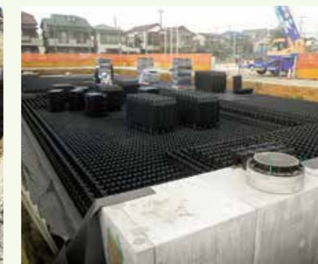
Elementary school in Chiba Prefecture 460m 3
